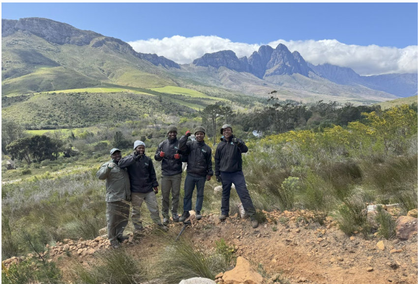
Serious repair work done on the Goddess Trail in Botmaskop (left). The team working hard on Stellenbosch Mountain (top).
